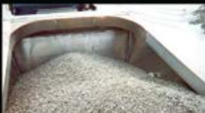
Large radius gussets on bulkhead
