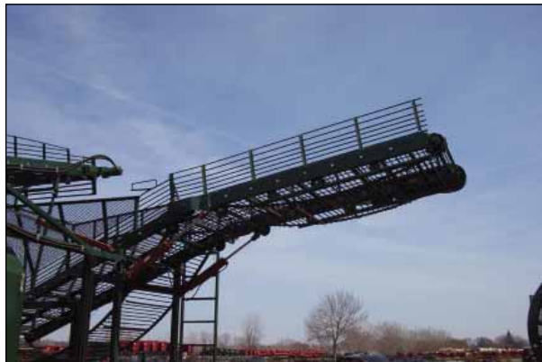
Figure 74. – Truck Boom Conveyor
